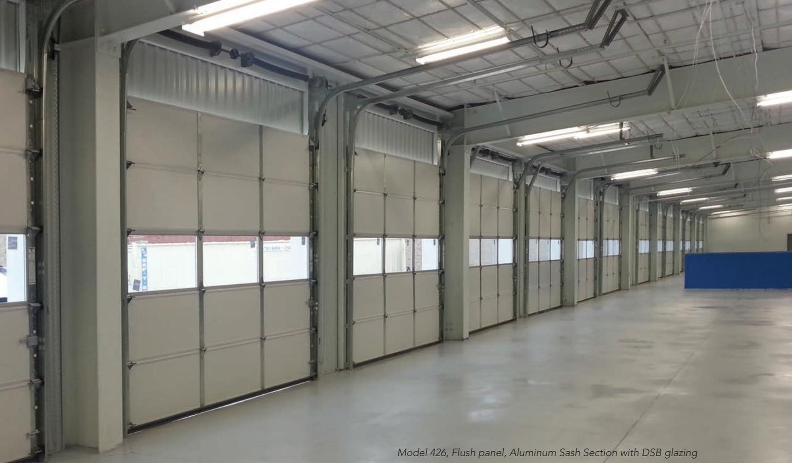
Model 426, Flush panel, Aluminum Sash Section with DSB glazing
